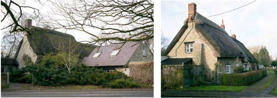
Small landmarks or 'marker' buildings are created where gables front the street (Hazel Cottage and Bramble Cottage, above)
