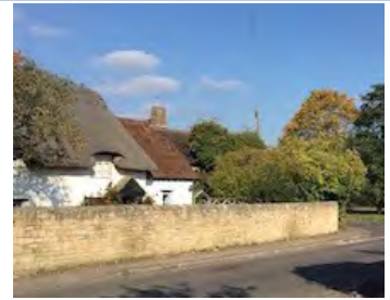
Typical stone boundary wall
