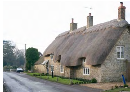
Example of building frontage set directly against public grass verge
